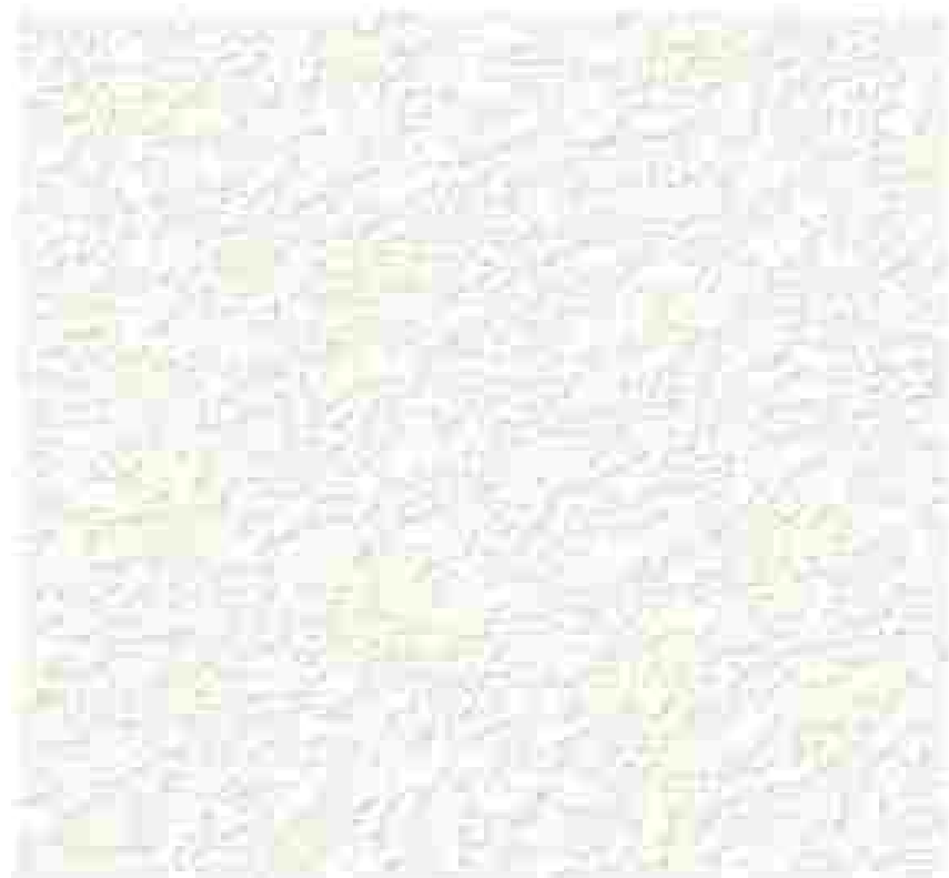
Item Plaster and Paint Area of use Exterior Facade
