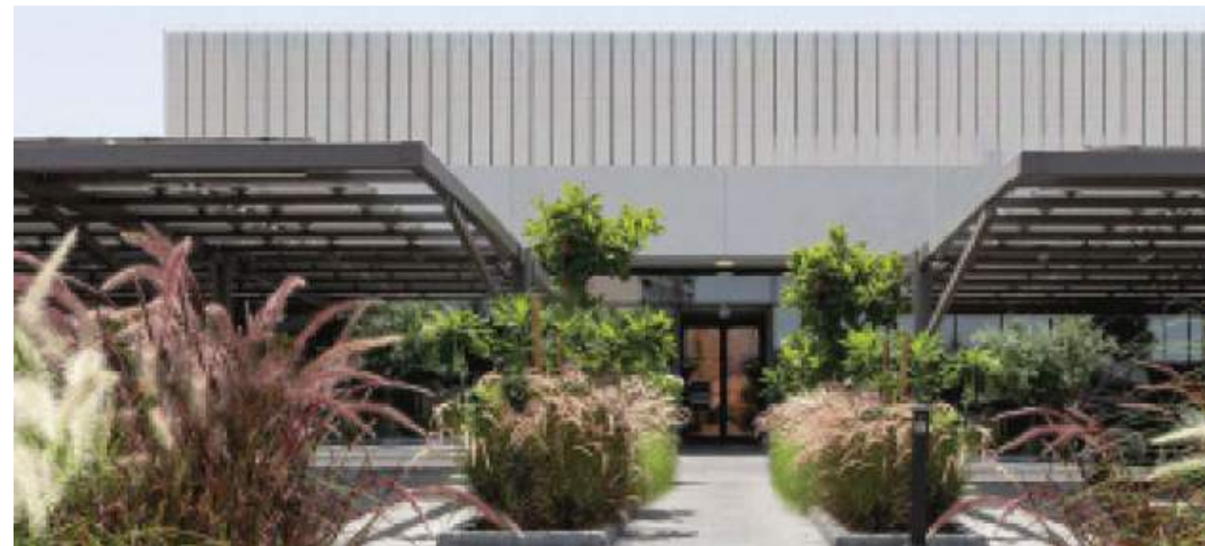
Figure 2.13 Community Facilities Images
