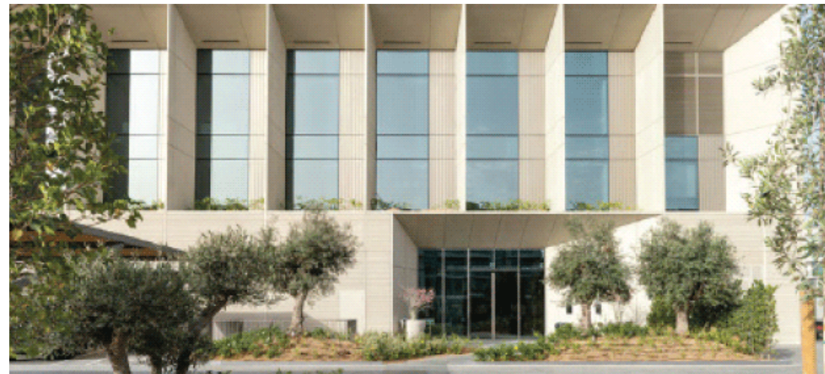
Figure 2.13 Community Facilities Images
